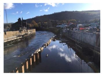
Reinstatement next to Burnley Road is almost complete. The area includes flood glass installed in the wall, stone paving, resin bound sections, a tree planter, bench and refuse bin (photo left).
